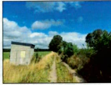
Plate 2 15m hedgerow section (right) at entrance to temporary construction compound – proposed for removal
