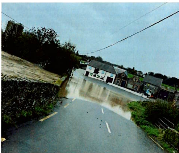
Fig. 17: October 23, 2023 Flooding (Storm Babet)
